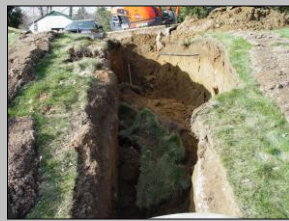
Shear Wall Failure
